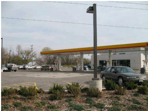
Photo 8 - 45: Southeast corner of Carlisle Road and Highway 6
